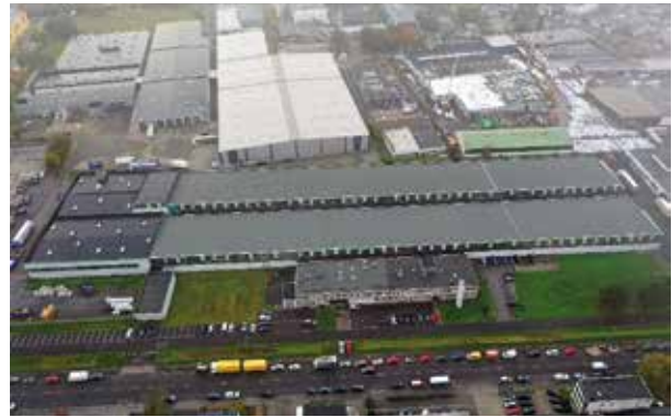
The warehouse is 265 m in total
