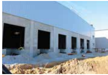
Loading ramps are levelled for lorry loading
