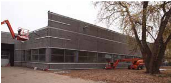
The new façade cladding is installed
