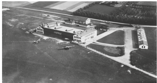
Flight operations ceased around 1950 and the buildings were demolished, creating new space for housing and businesses
