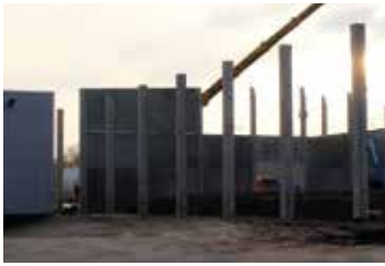
Support pillars and walls are built
